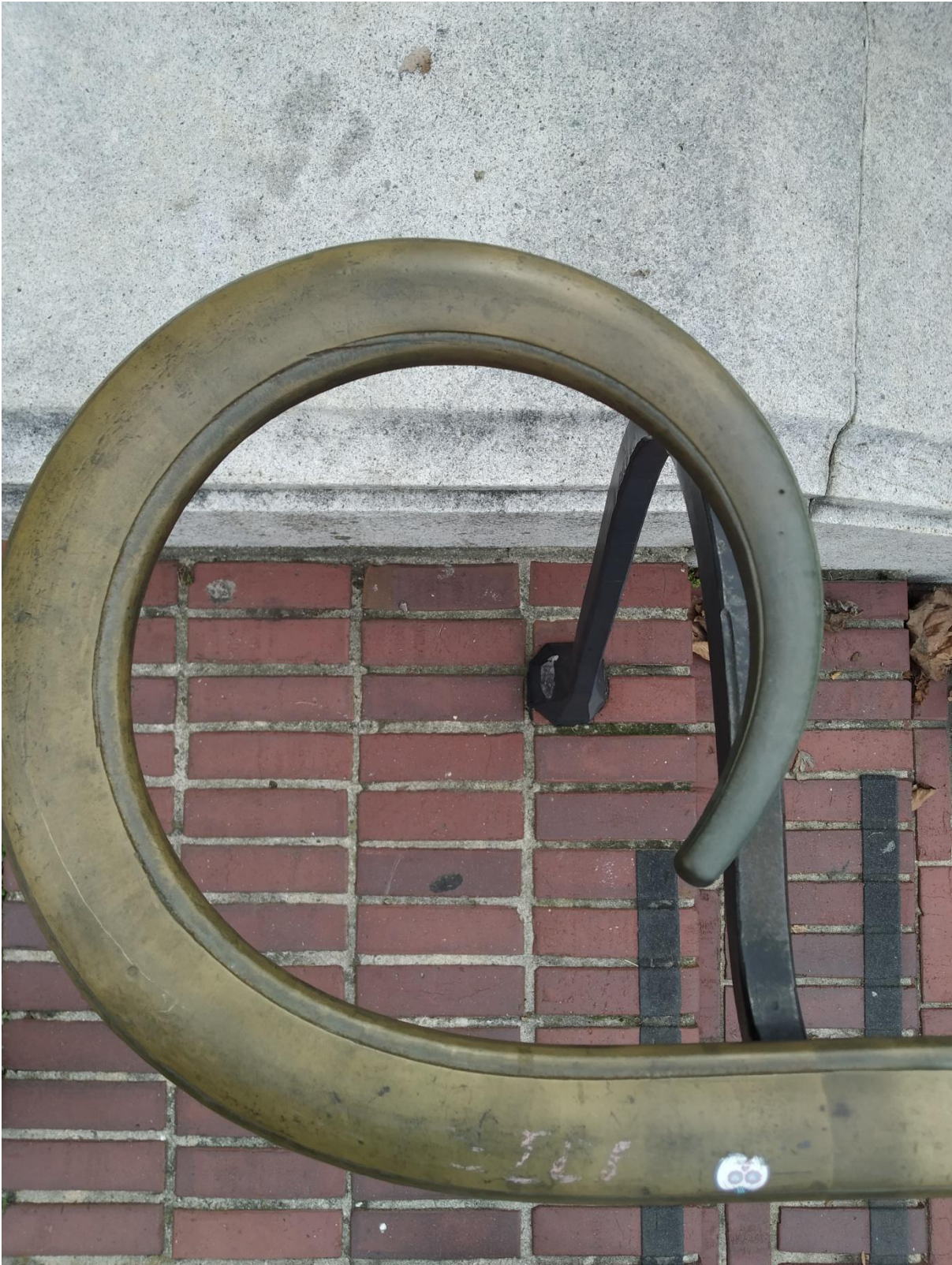
Exterior detail from UC Berkeley campus
