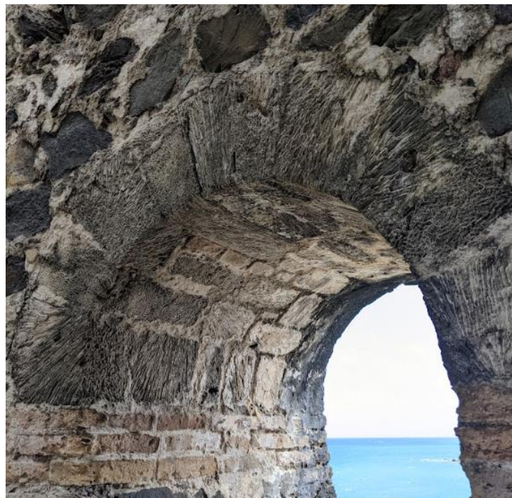
Figure 35 Shaped coral is featured in various structures at Estate Coakley Bay. This image depicts ‘shaped’ coral blocks used in the openings in the site’s wind-powered sugarmill (Zahedi 2021).
