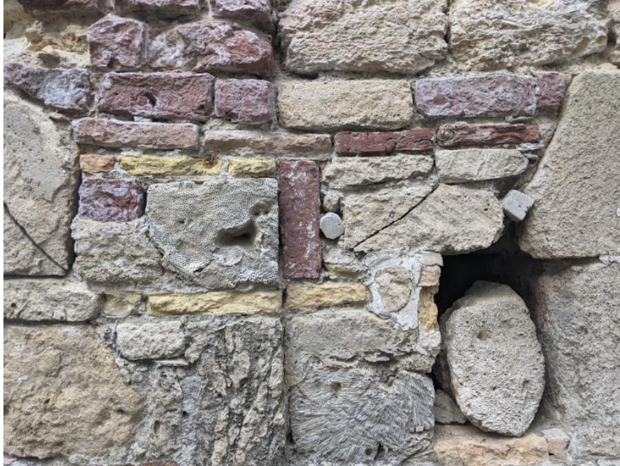
Figure 23 A structure in Christiansted built with a combination of several species of coral, brick, and locally quarried stone (Zahedi 2020).
