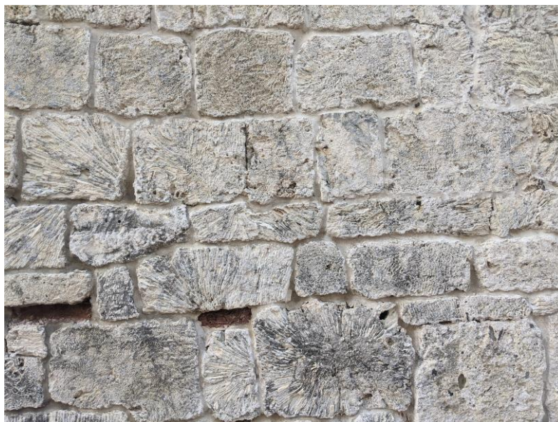
Figure 37 Wall constructed entirely of Pseudodiploria strigosa that has been shaped into blocks (Zahedi 2020).
