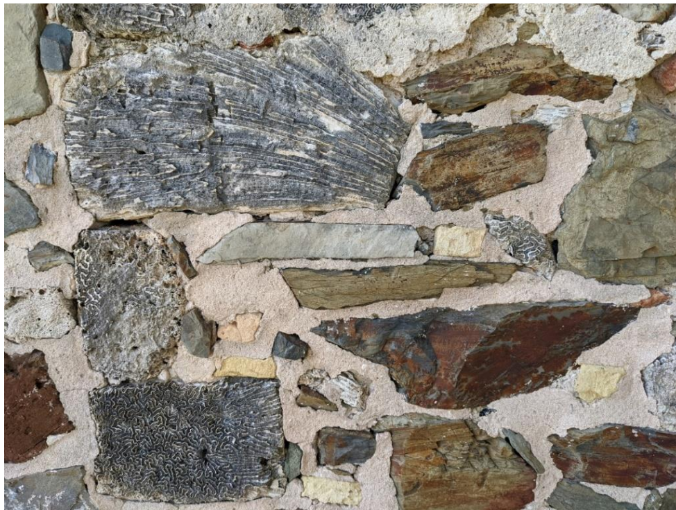
Figure 32 The masonry style at Estate Great Pond features coral, blue bit, and brick fragments (Zahedi 2020).
