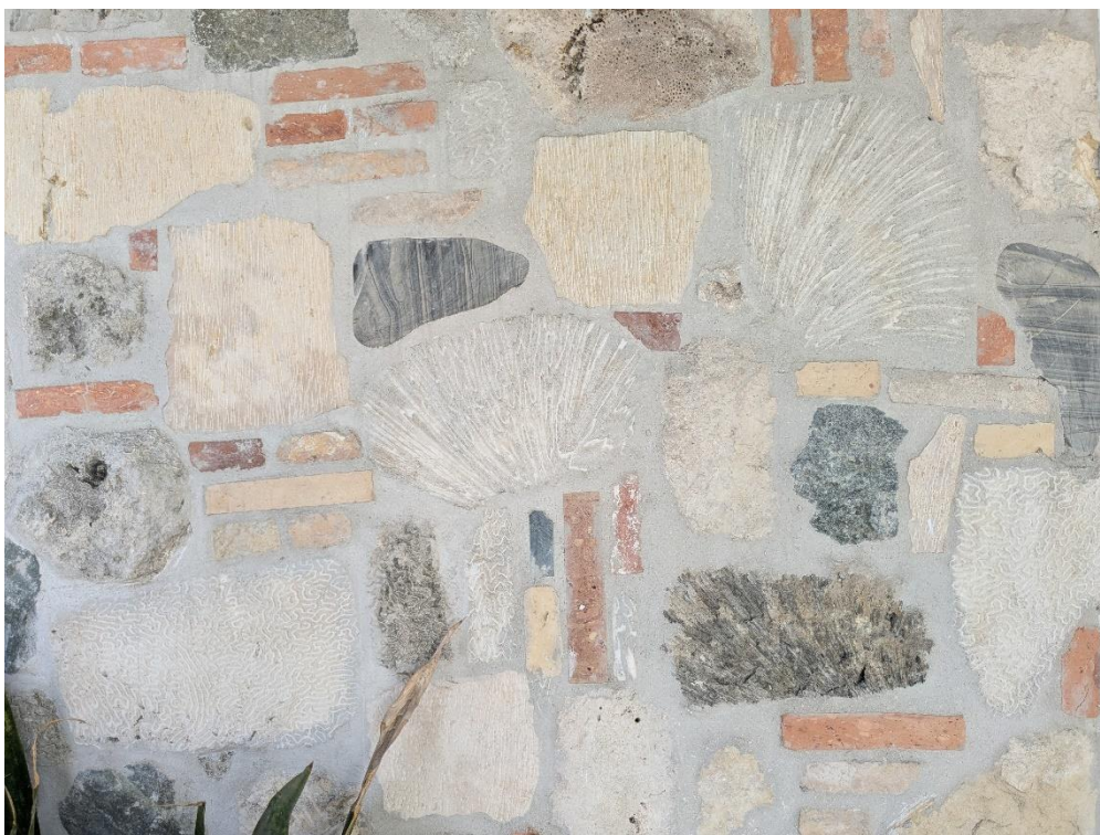
Figure 42 Repurposed coral blocks which have been sliced into thin veneers to preserve the historic aesthetic whilst adhering to contemporary building and environmental codes (Zahedi 2024).
