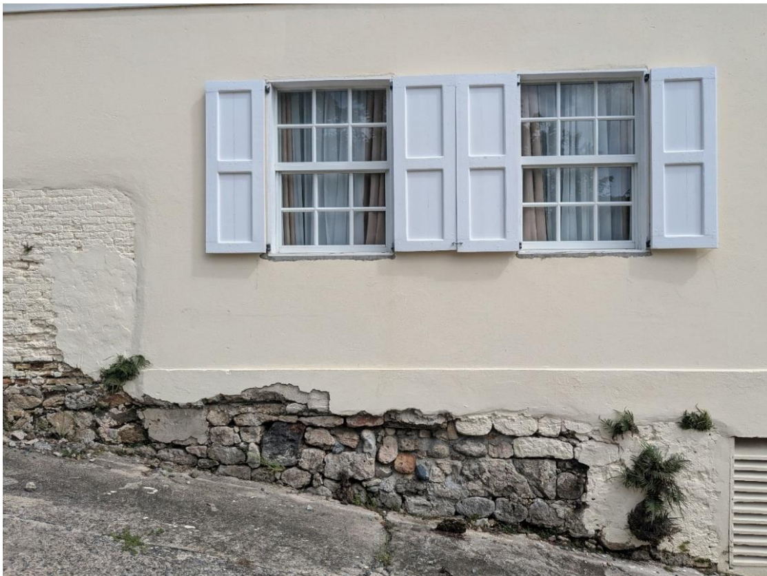
Figure 15 A partially exposed coral foundation in Christiansted (Zahedi 2023).
